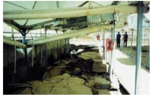
Concrete foundations washed away by running water
